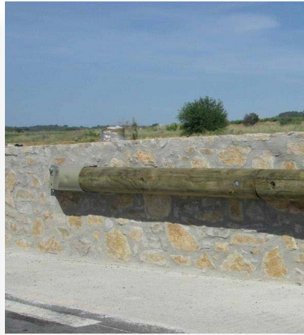
G/G+ Transition on concrete wall 800 460
