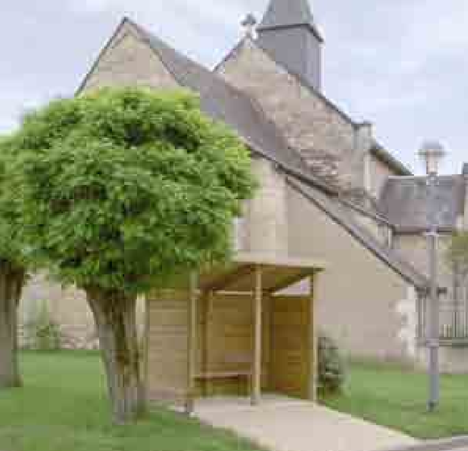
627 510 abri bus sciage marquesina traviesas bus shelter - sawing
